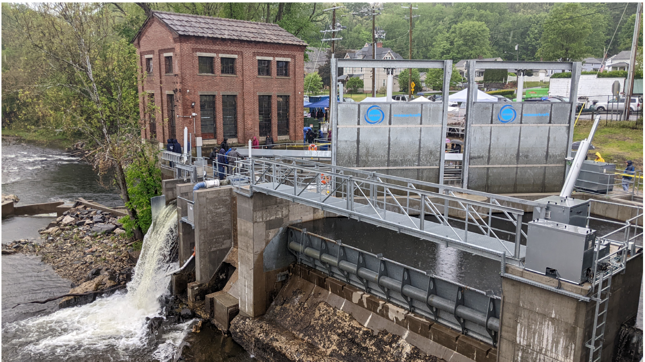
A view of the Upper Collinsville hydropower plant on the Farmington River in Canton, CT.
